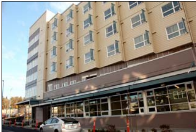
Photo courtesy of the Low Income Housing Institute [enlarge]
